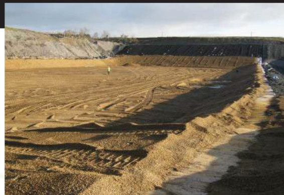
Placing the granular leachate drainage blanket
