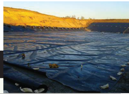
Laying and welding the HDPE geomembrane
