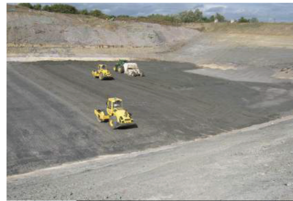
Compacting the clay liner
