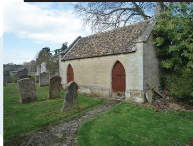
Exton Church Toilet and Kitchenette
